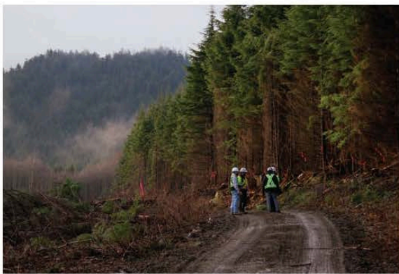
Work crews survey the pipeline right-of-way area.
